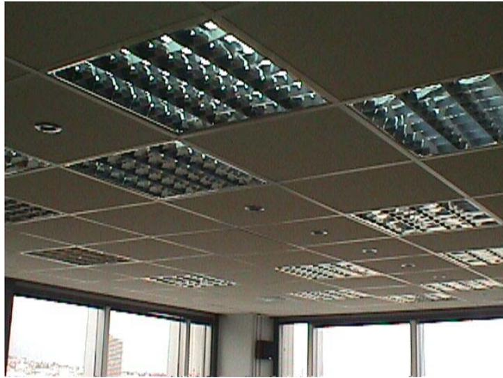
**Luminaires near the façade. Their control can be separated from the control applied to the luminaires located at the core of the building.**
